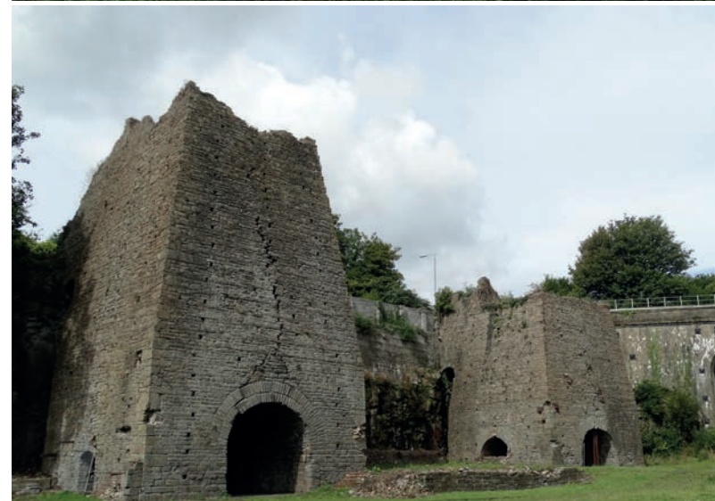
The work of dedicated volunteers who cleared vegetation from the Blast Furnaces at Neath Abbey Ironworks.
